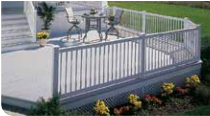
DECKING AND RAILING
